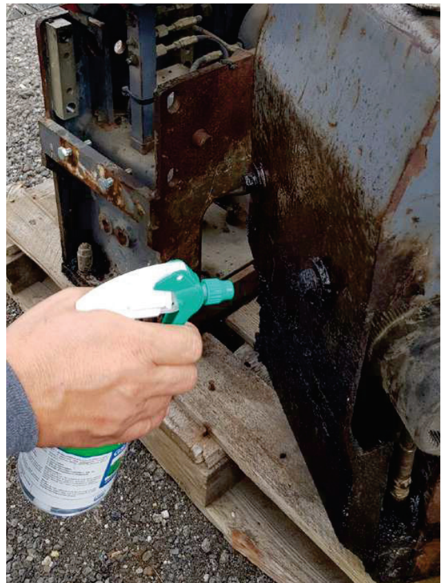
Removing bitumen with GS 200
