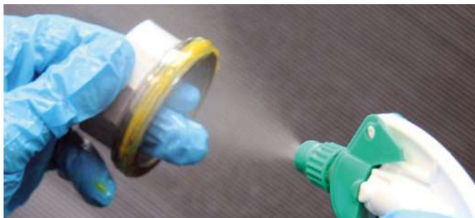
Removing sealant with GS 200
