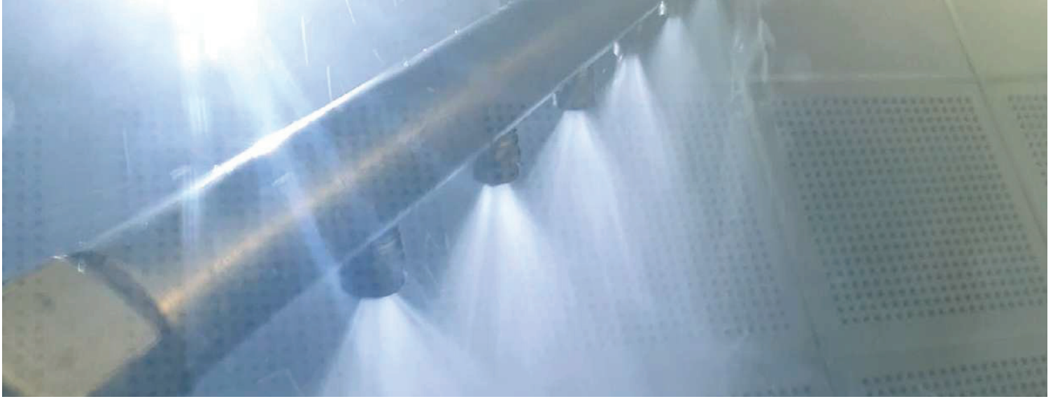
Mechanical cleaning in the HTW
